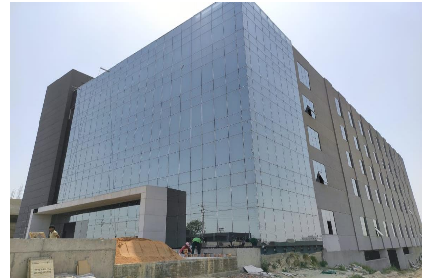
Site Pictures: Block I at Plot No 10, Sector 156, Noida, Gautam Budh Nagar, Uttar Pradesh
